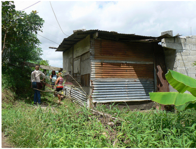
House, Panama City, Panama, photo by Wes Janz, 2008
